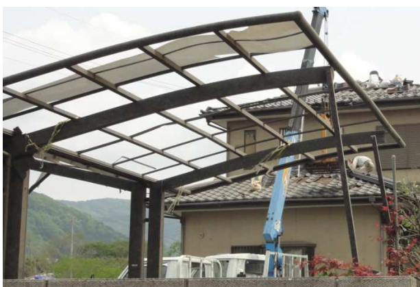
DOD = 1 Debris-related destruction of roofing panels Courtesy of Wind Engineering Research Center, Tokyo Polytechnic University
