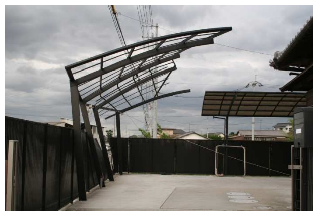
DOD = 2 Wind-related inclination of frames (Application of UB to a three-column cantilevered carport without walls) Courtesy of Institute of Technology and Science, Tokushima University
