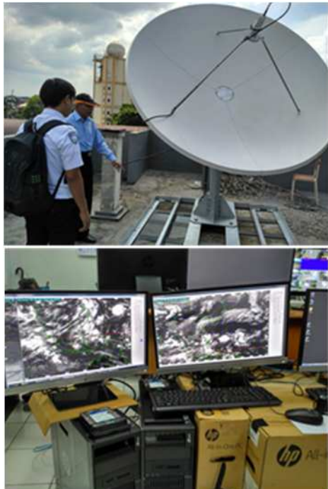
Figure 2 Reception antenna (top) and computer clients (bottom) of HimawariCast installed in BMKG's college
